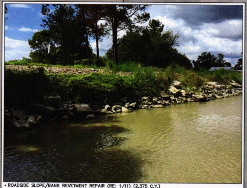
• ROADSIDE SLOPE/BANK REVETMENT REPAIR (RE: 1/11) (2,375 C.Y.)
