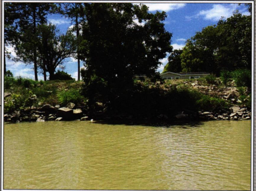
• ROADSIDE SLOPE/BANK REVETMENT REPAIR (RE: 1/11) (476 C.Y.)
