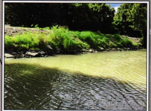
• ROADSIDE SLOPE/BANK REVETMENT REPAIR (RE: 1/11) (95 C.Y.)
