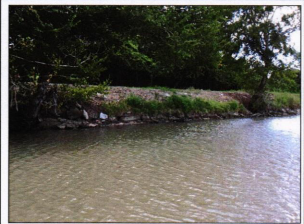
• ROADSIDE SLOPE/BANK REVETMENT REPAIR (RE: 1/11) (305 C.Y.)
